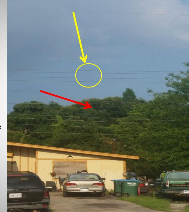
This 230 circuit is a bundled conductor circuit and the top four wires were actually the bundled top and middle phases.
